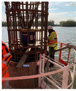
Installation of O-Cell and reinforcing cage
