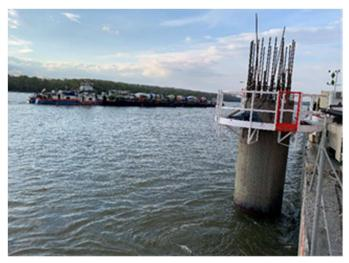
Concrete wagons on a barge ready for their delivery into the pile in the middle of the river
