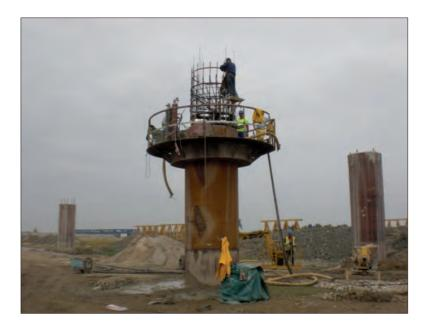
Installation of O-cell test pile
